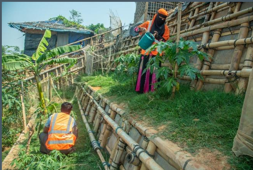
Above: Women and men volunteers worked together to build and grow vegetation on slope stabilisers in refugee camps in Cox's Bazar. Source: Australian Humanitarian Partnership
